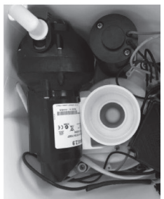
15. Replace rinse pump & control box
